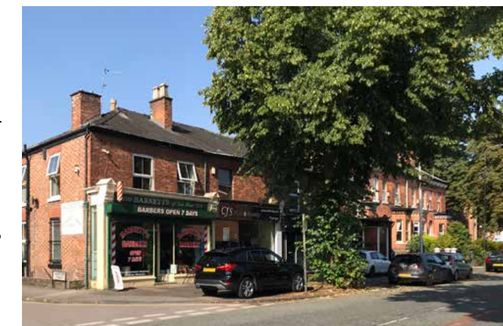
Figure 5: Retail units on Northenden Road
