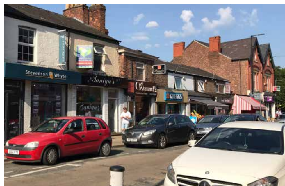
Figure 50: Retail units on Northenden Road
