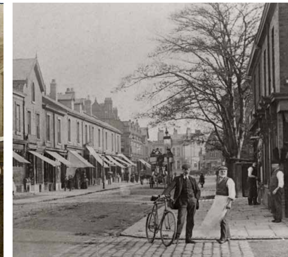
Figure 9: View east along Northenden Road towards the Legh Arms circa 1910, source: Trafford Lifetimes
