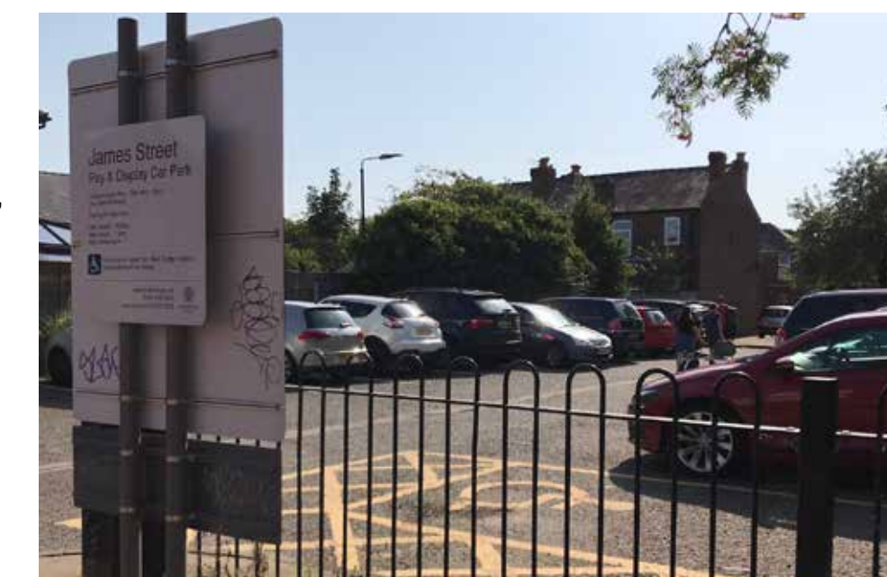
Figure 6: Surface level car park at James Street
