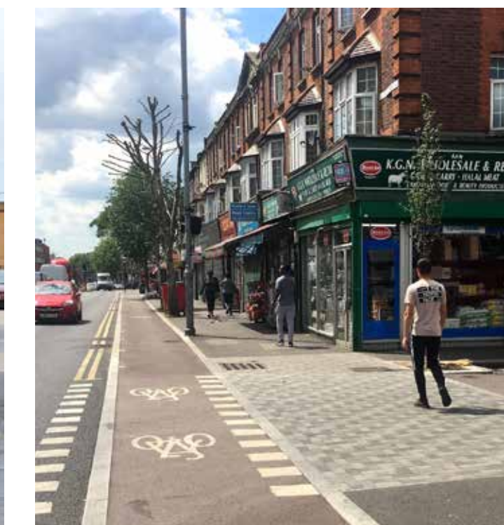
SIDE STREET CROSSINGS IMPROVED
