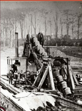
Construction of the Manchester Ship Canal
