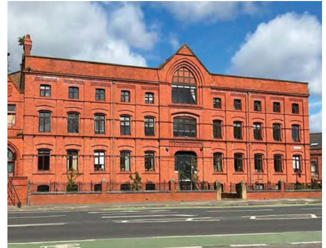
Strong parapet line interrupted by a gable with pitched roof behind.
