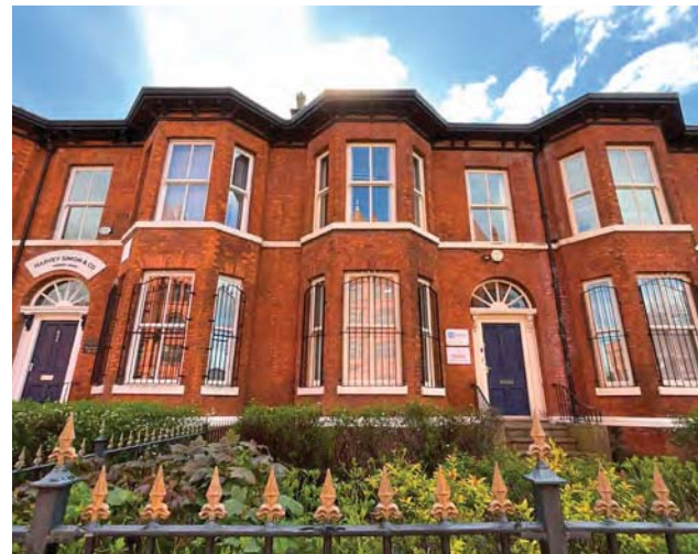
Double-storey bays at Trafford Place.
