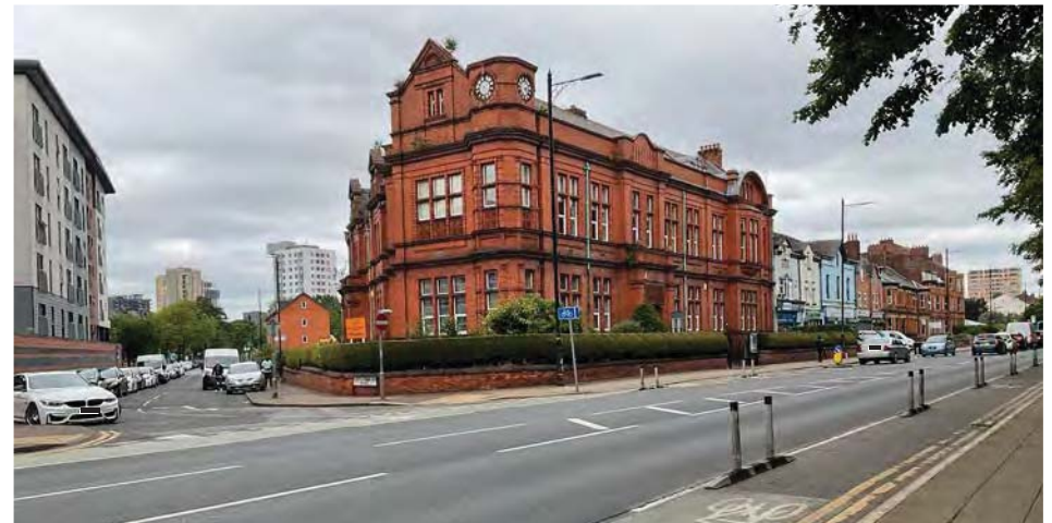
2.12 View I, looking west through the proposed extension and east along its edge
