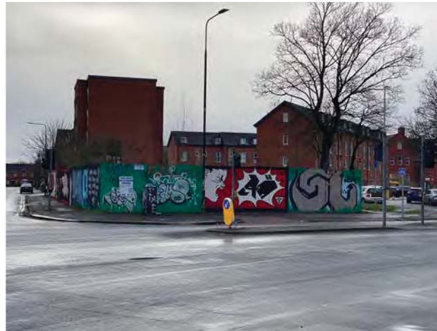
4.51 Northumberland Road gap site and modern town house and apartment block development behind
