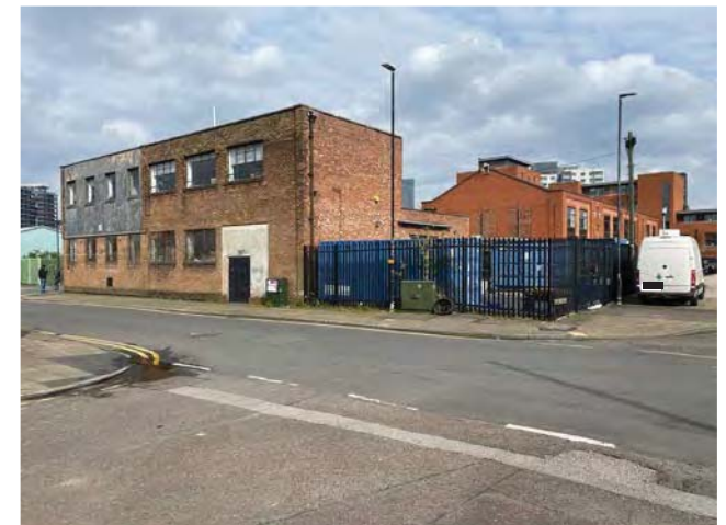
7.6 Poor quality redevelopment to Hadfield Street following the loss of terraces
