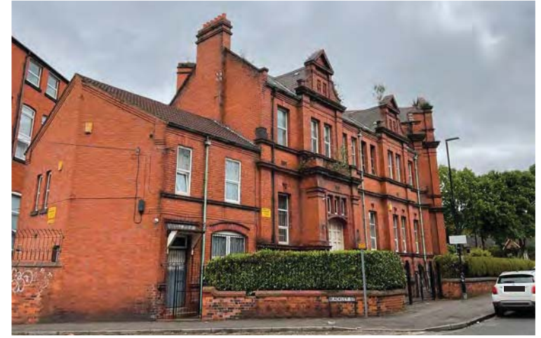
8.11 Former Technical Institute, Northumberland Road frontage
