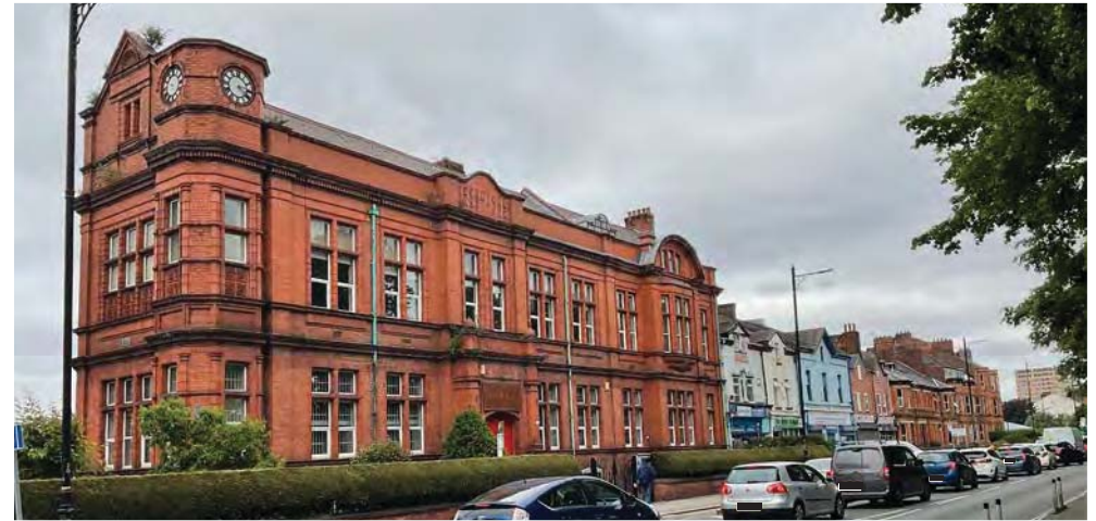
2.13 View I, looking east along the proposed extension
