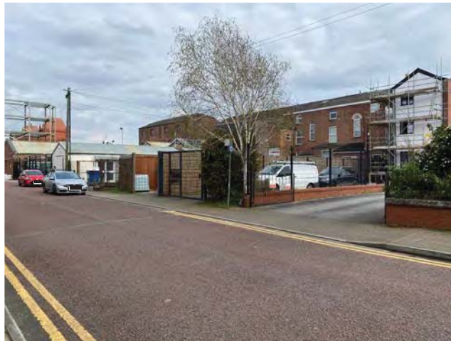
4.42 Rear elevations of Dover Terrace and Almondbury Place, with detracting features
