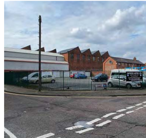
5.14 Views over the industrial belt include important industrial sawtooth roof forms
