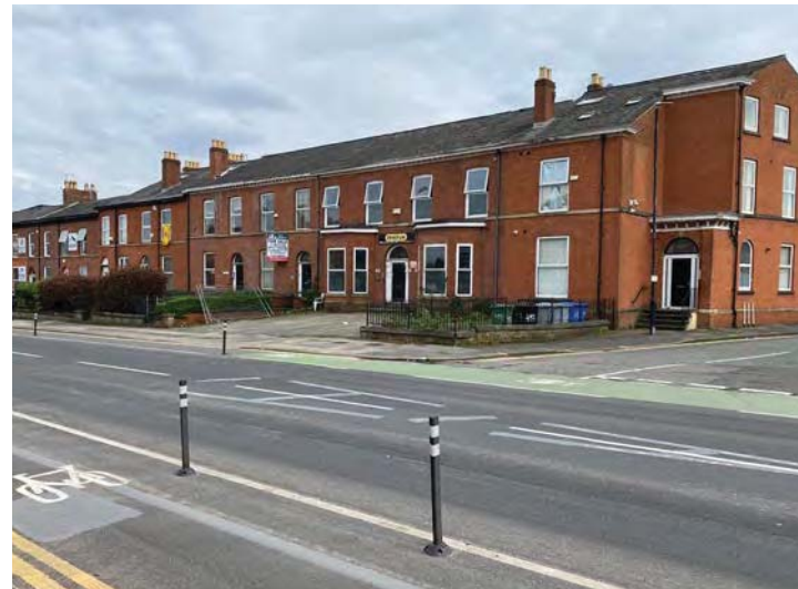
7.3 Changes to windows, and a rebuilt end bay, to Winfield Terrace
