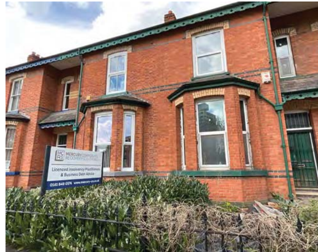
Single-storey bays at Birkdale Terrace,
