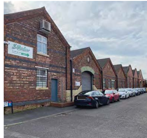
5.6 Linear views along Turner Street frame the highly characteristic articulated gables
