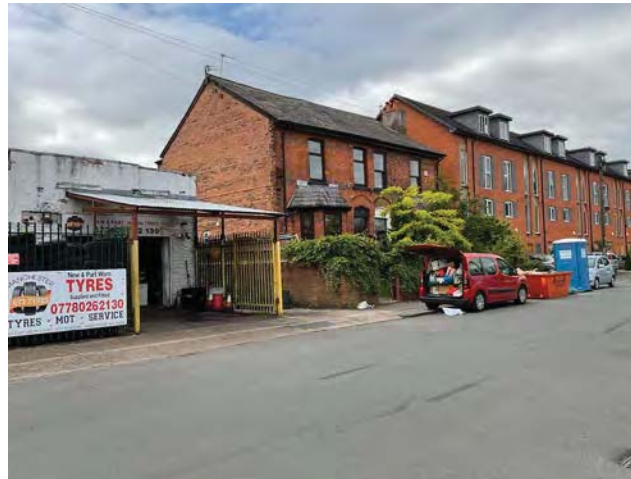
4.57 East Union Street garage and nos. 18-20
