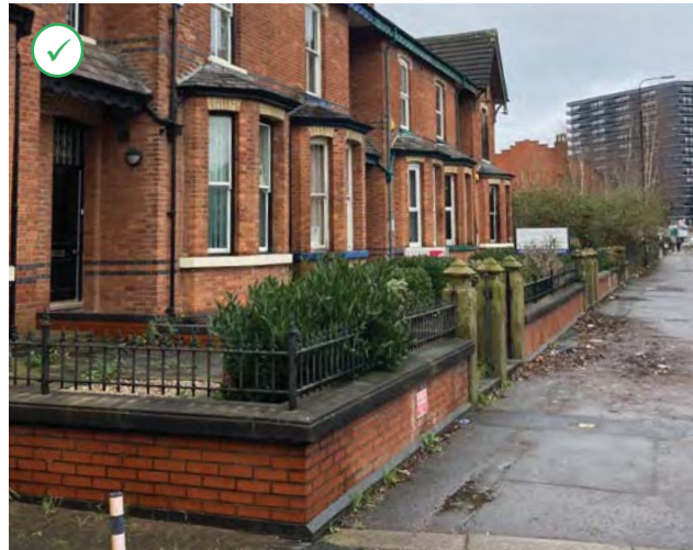
Example of continuous front garden boundary wall along Chester Road
