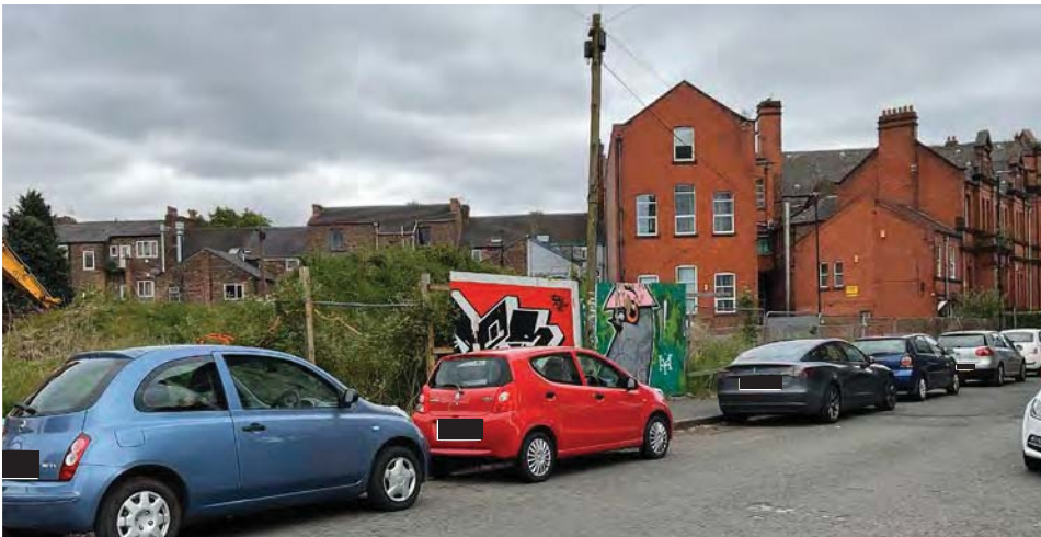
8.12 Former Technical Institute, rear (gap site behind)
