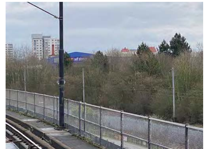
6.2 View from Pomona Metrolink station (zoomed in to identify the relevant features)
