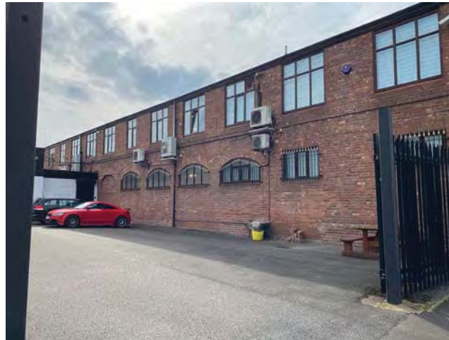
4.21 Old Engine House, Lund Street
