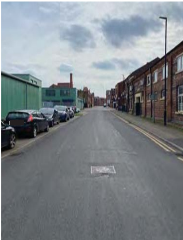
5.4 Views south on Hadfield Street hint at the important commercial cluster within the conservation area whilst revealing the Empress Brewery chimney
