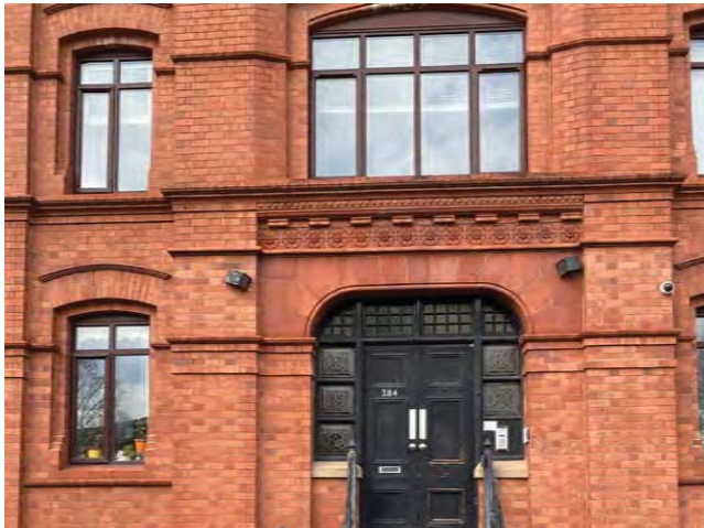
4.11 Fine door joinery and detail at 384 Chester Road
