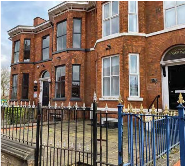
4.36 Canted bay detail at Trafford Place
