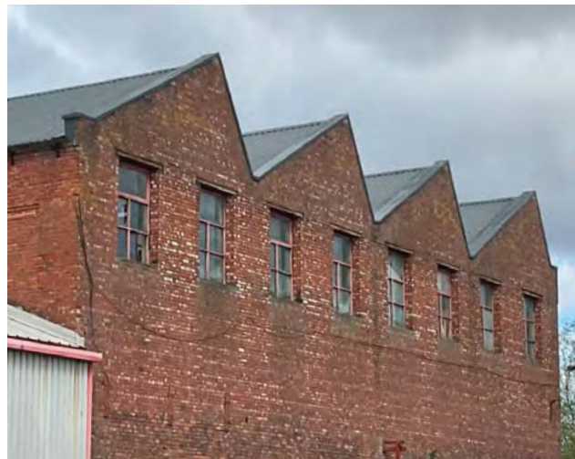
Sawtooth roof at Former Empress Machine Tool Works.
