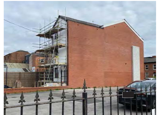
4.40 Rebuilt end gable of Dover Terrace
