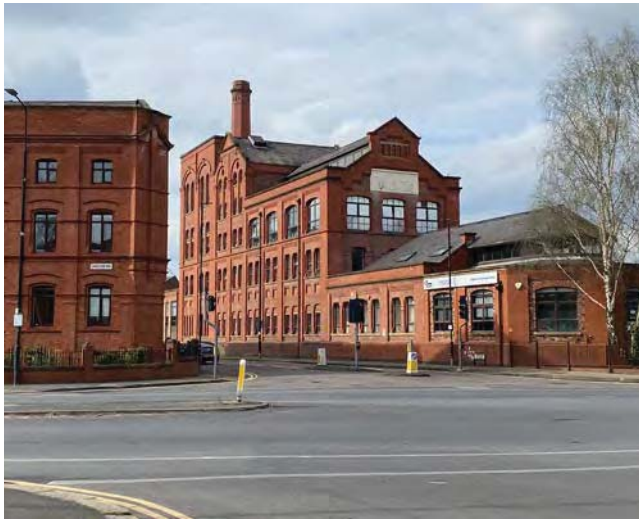
5.9 Key landmarks, such as the Empress Brewery dominate the junction of Chester Road and Northumberland Road
