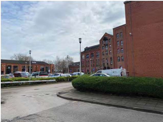
4.9 Empress Brewery, site interior with historic and modern buildings
