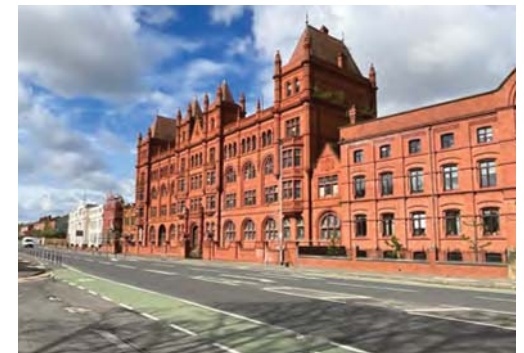
The Essence Factory, Chester Road.
