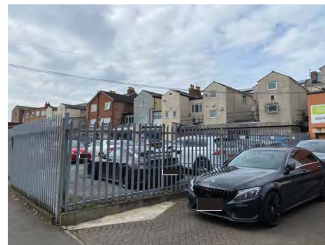
7.1 Loss of gardens, and alteration to rear elevations along Winfield Terrace
