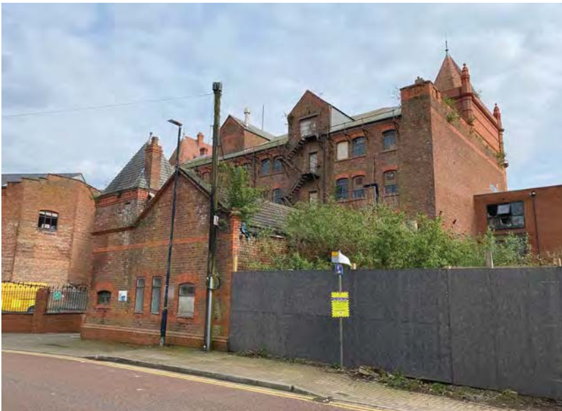
4.4 Rear elevation and outbuildings to the Essence Factory, all Grade II listed, Wright Street
