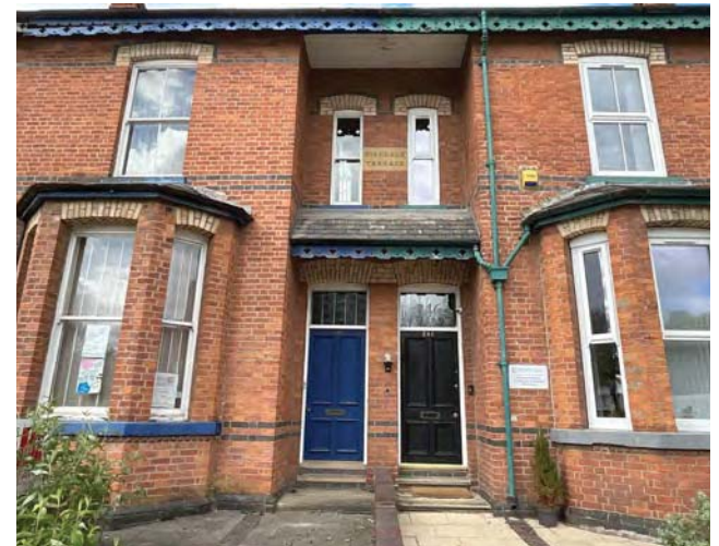
Recessed bay at Birkdale Terrace.
