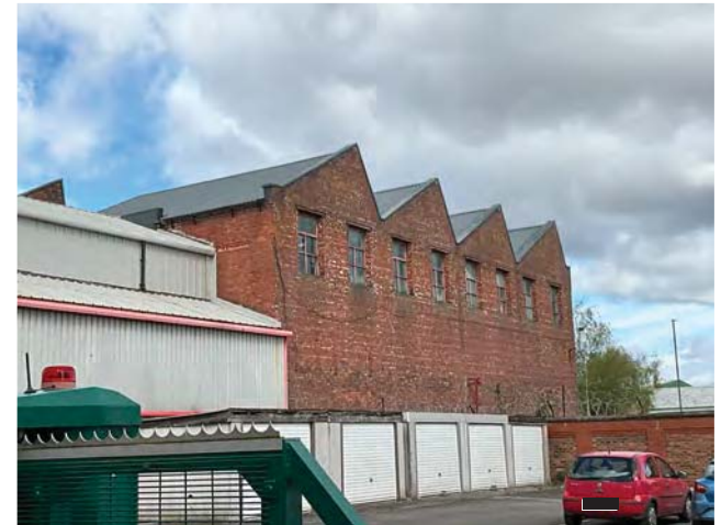
Sawtooth roof at Former Empress Machine Tool Works
