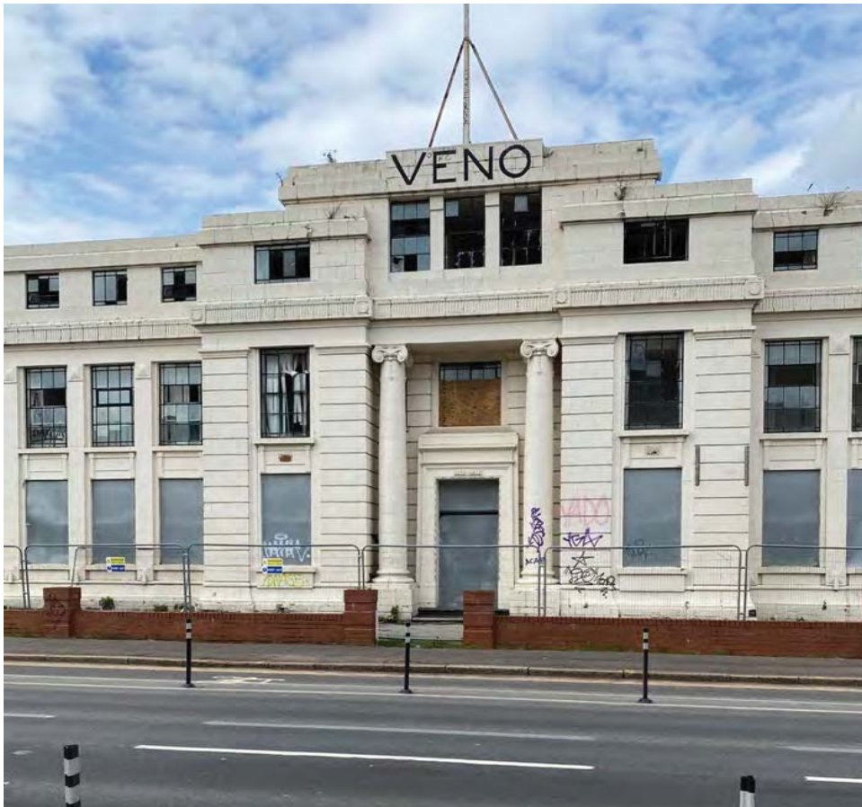
7.10 Deterioration and Heras fencing to the Venetian Building
