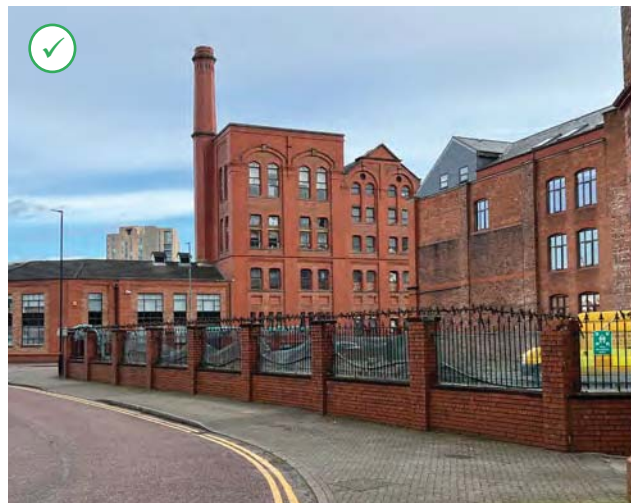
Example of mill building wall with fence along Wright Street
