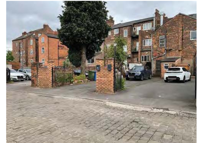
4.52 Rear of houses to Stretford Road
