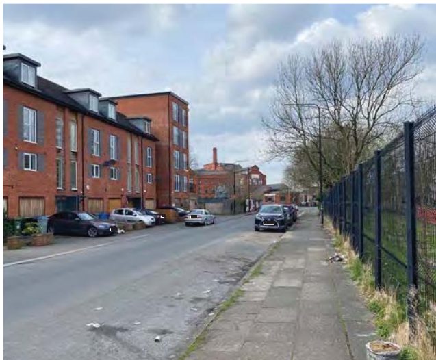
6.13 Empress Brewery, including the chimney, becomes increasingly prominent moving west on East Union Street
