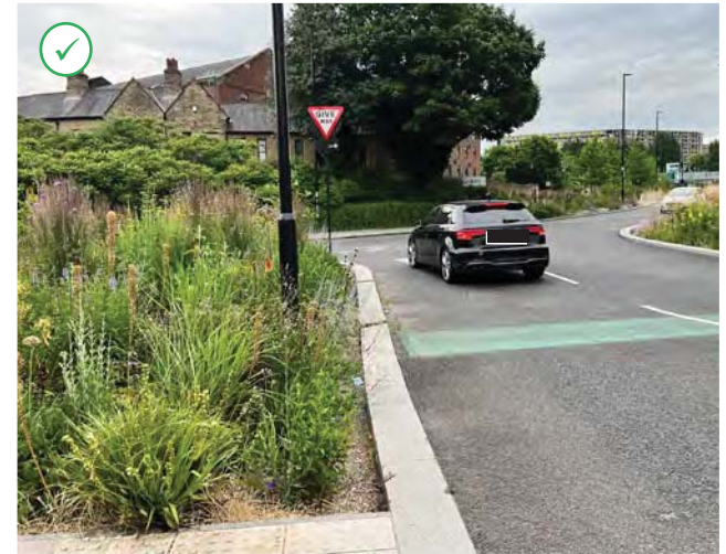
Example of planted bioswales as part of SuDS
