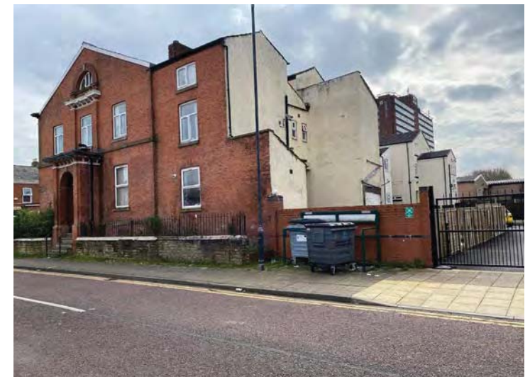
7.4 Poor quality rear elevation and land to Dover Terrace
