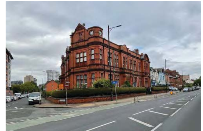
2.23 Mixed modern built form to the west, north and northeast, visible beyond the former Technical Institute
