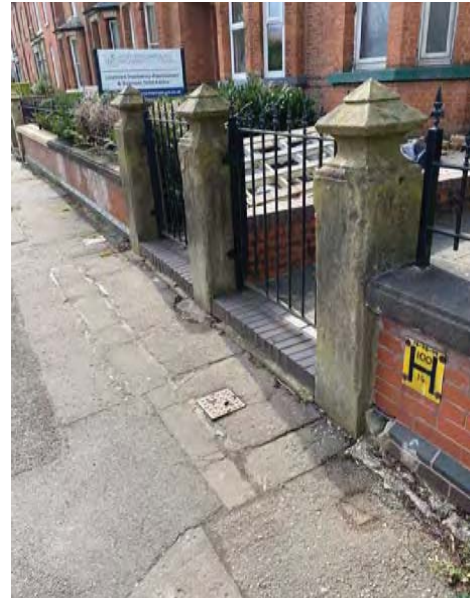
4.31 Historic gatepiers at Birkdale Terrace
