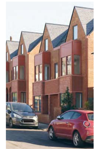
Precedent- Keelson Yard by 31/44 Architects
