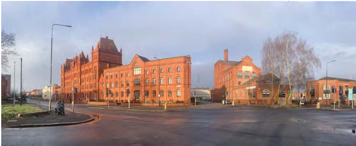
2.10 View K, west, southwest and northwest into the conservation area
