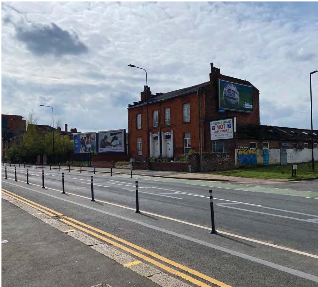
6.8 The northern gateway is marred by advertisement hoarding and the current condition of Cornbrook Terrace
