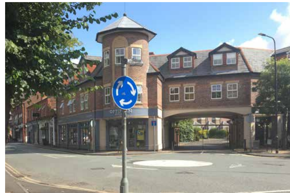
Figure 5: Modern retail and residential units on Victoria Road
