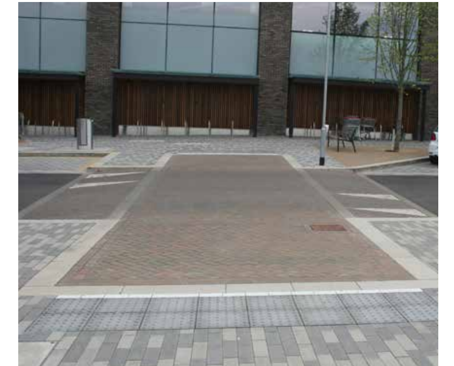
RAISED TABLES MARK VILLAGE ENTRANCES & 20 MPH ZONE
